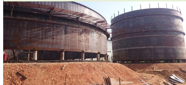
Fabrication of Storage Tanks, Gulbarga
